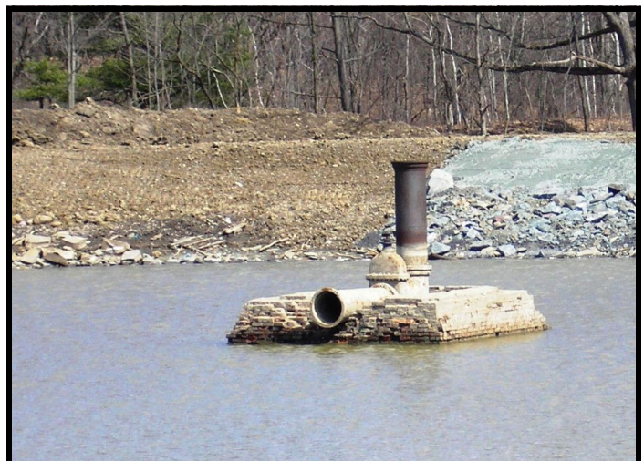
Original Stand Pipe, c. 1877, at Watervliet Reservoir on Watervliet Shaker Road (Rte. 155).
