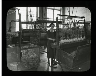
Yarn from spinning bobbins was reversed and tightened to a second bobbin and then wound onto larger 'Warp Spools.'
