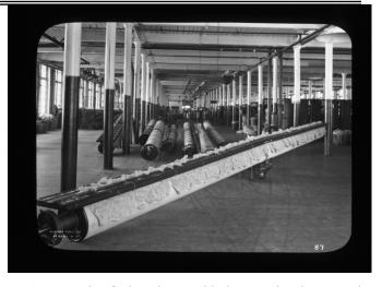
An example of a long beam with the completed warp ends within the harness nettle to be sent to a large loom for weaving.
