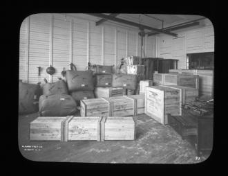
Finished felts of various sizes ready to be shipped. Domestic felts were wrapped in heavy paper and cloth bags. Wooden crates were used for exports.
