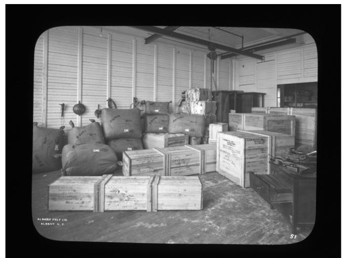
Finished felts of various sizes ready to be shipped. Domestic felts were wrapped in heavy paper and cloth bags. Wooden crates were used for exports.
