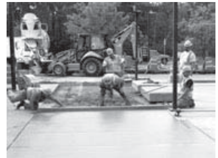
Photos from our recent plaza and parking lot reconstruction.
